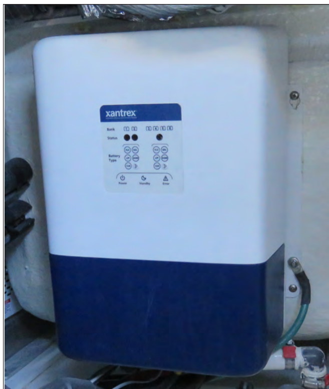
Typical Battery Charger
