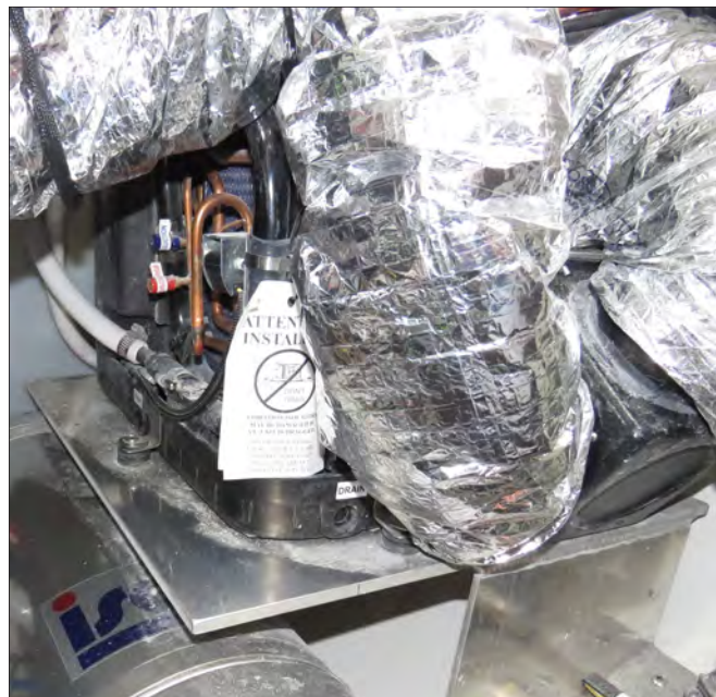
Typical Cabin Air Conditioning Unit & Condensation Pan Drain
