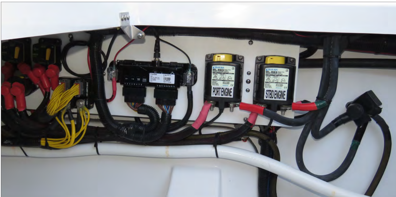
Engine Battery Switches In Aft Systems Compartment
