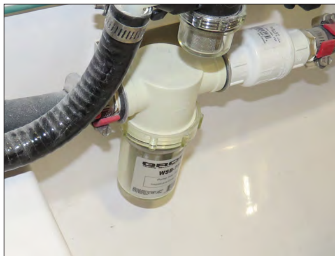
Typical SeaKeeper Pump Sea Strainer
