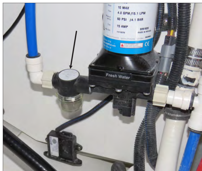
Fresh Water Pump & Strainer
