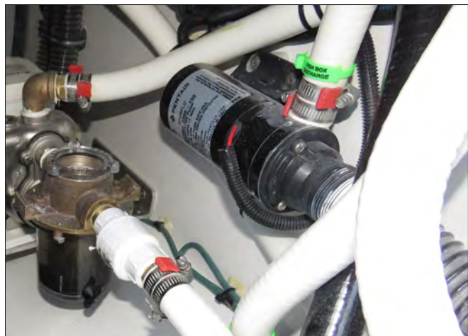
Aft Below Deck Fishbox Macerator Pump
